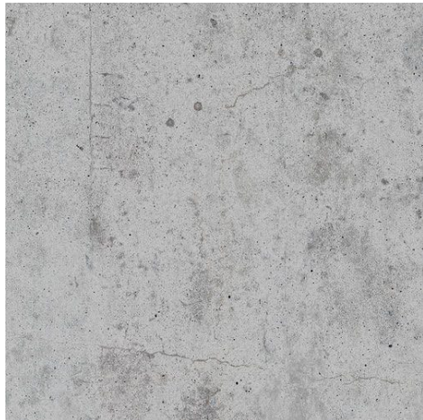
Polished Concrete Floor
