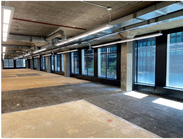
Open Exposed Ceiling
